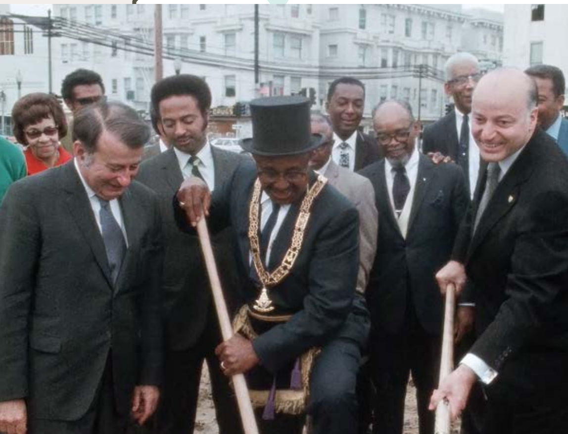
Prince Hall Grand Master Harry A. Brewer (center) is joined by Mayor Joseph Alioto (right) and Redevelopment Agency head Justin Herman at the groundbreaking for the Prince Hall Apartments in 1970.
